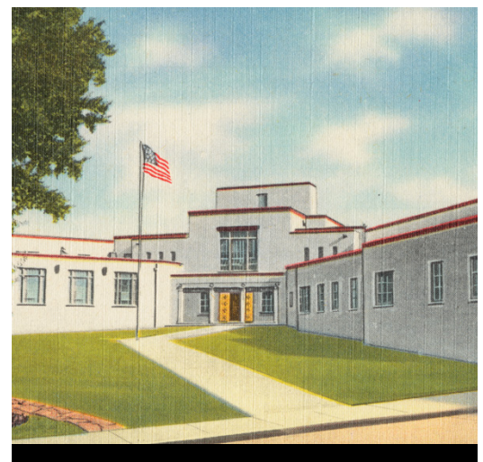
Supreme Court Building, ca. 1930-1945 (Boston Public Library)
